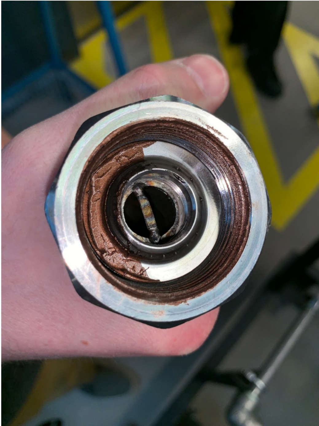
Figure 59 - Static Mixer within Pipe
